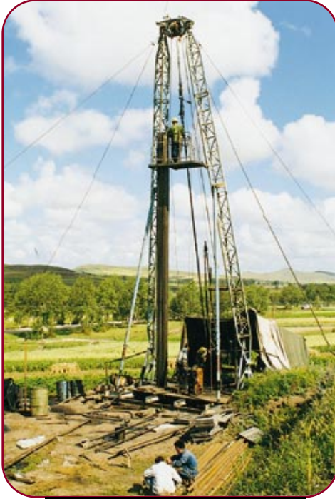
Drilling on Caijiaying project
